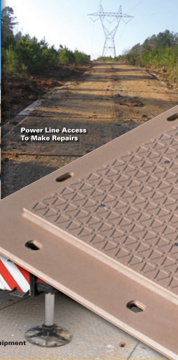
Transmission Line Construction In Tidal Marsh
