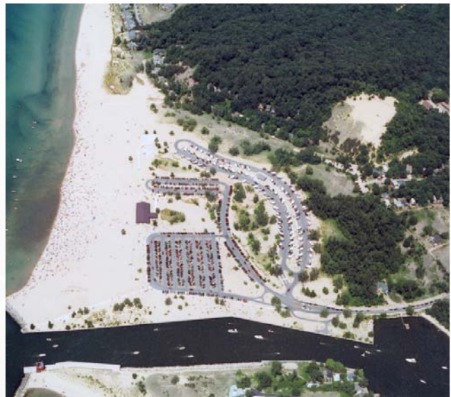
Holland State Park $4M Day Use and Campground Renovation
