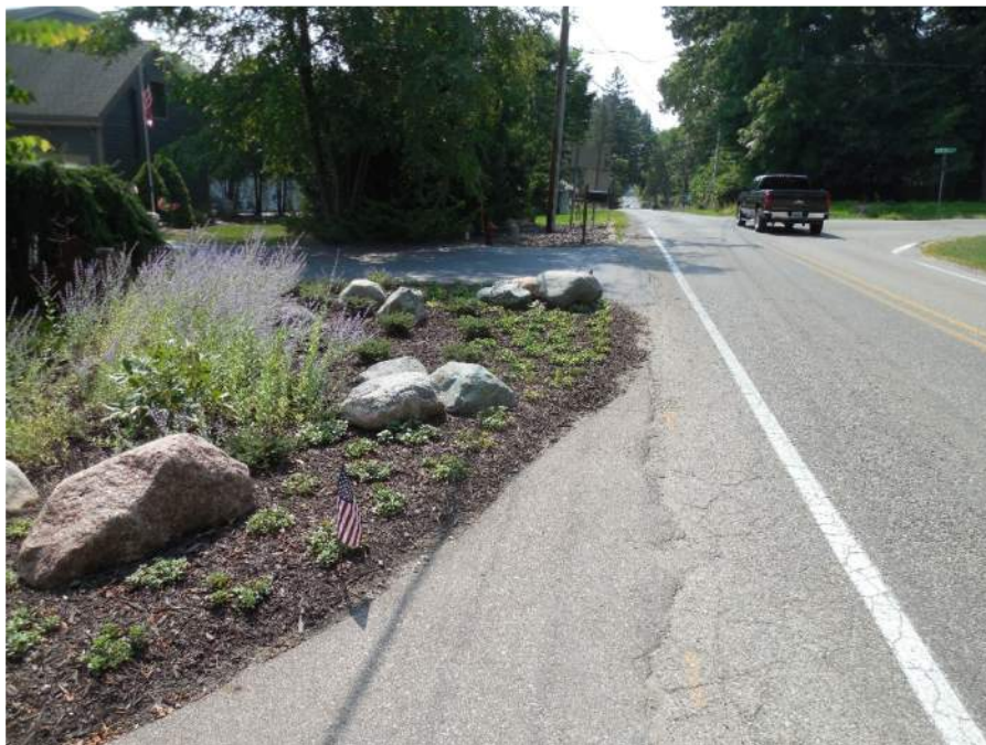
Photo 52: Landscaping at 5 Park Street Solution:
