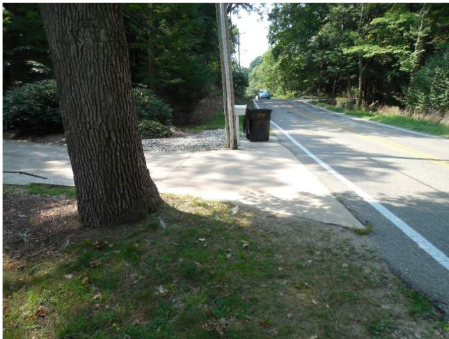
Photo 48: Pole at 107 Park Street, 5' clear from edge of asphalt
