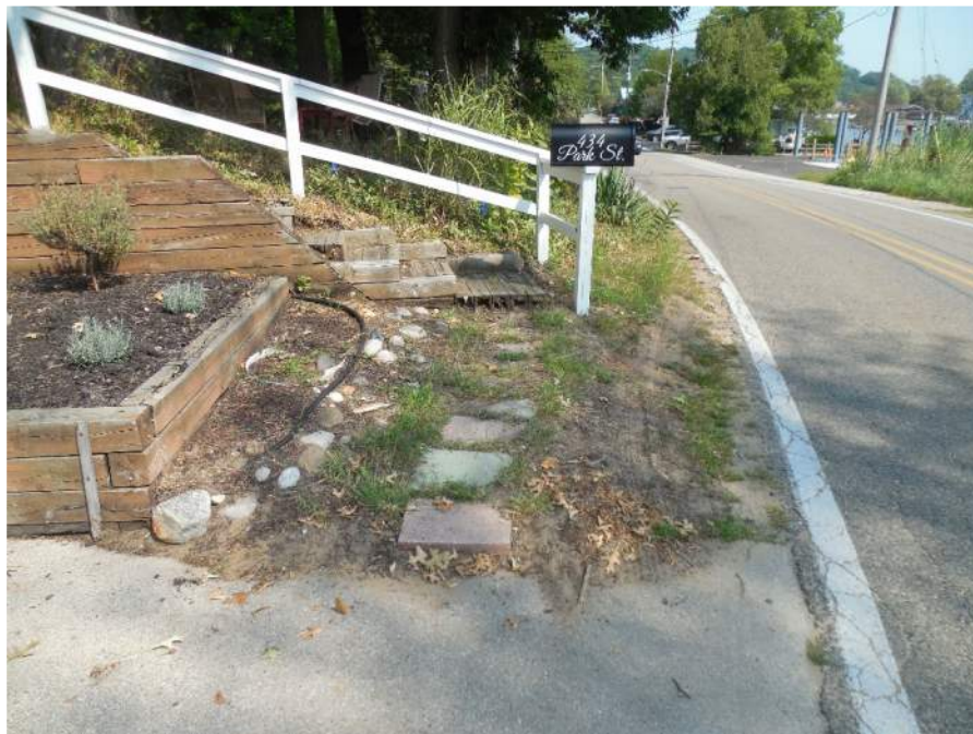
Photo 28: Slope and steps at 434 Park Street, north side of driveway
