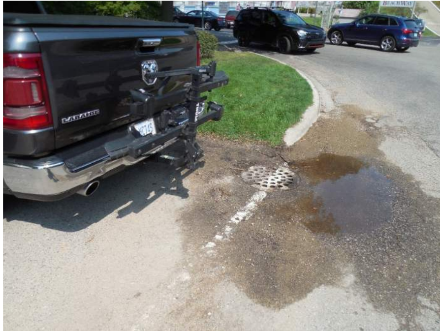
Photo 33: Catch basin at southwest corner of Park Street and Perryman Street
