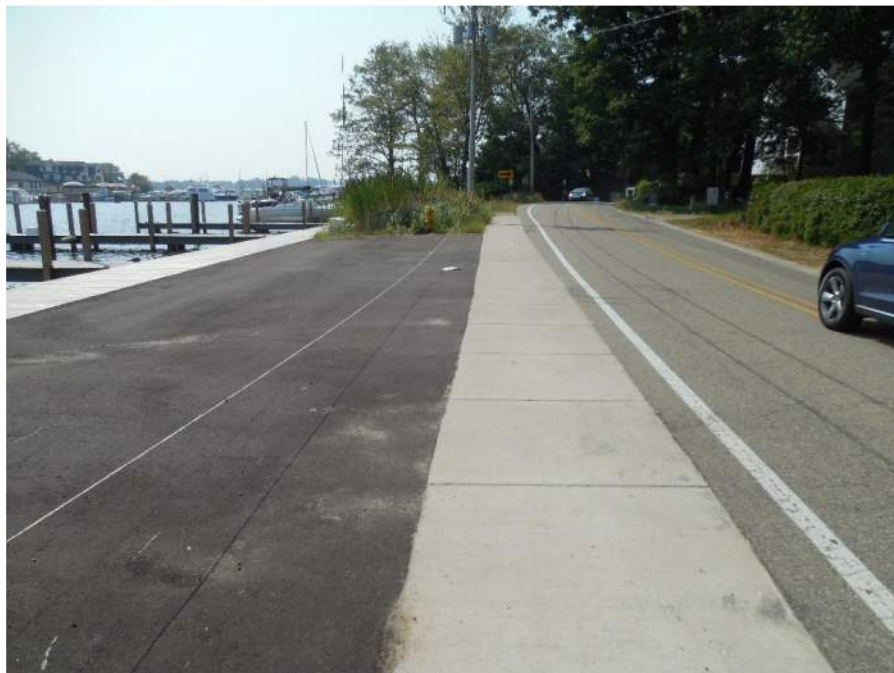
Photo 36: Existing sidewalk south of chain ferry Solution:
