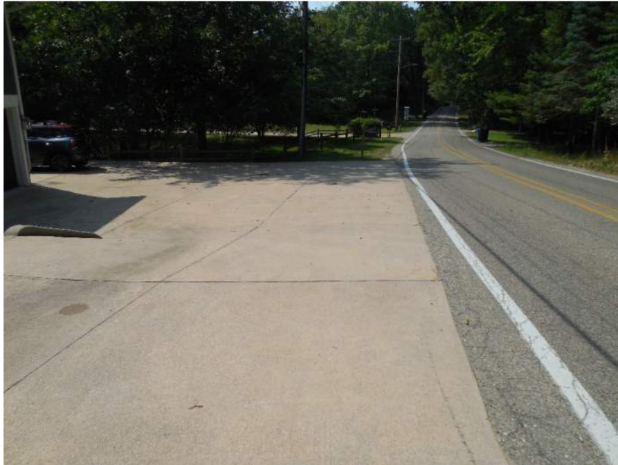
Photo 47: Driveway at 143 Park Street
