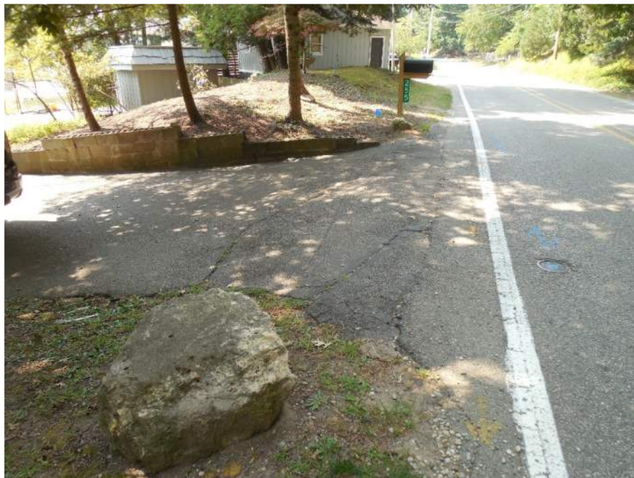
Photo 44: Driveway at 255 Park Street
