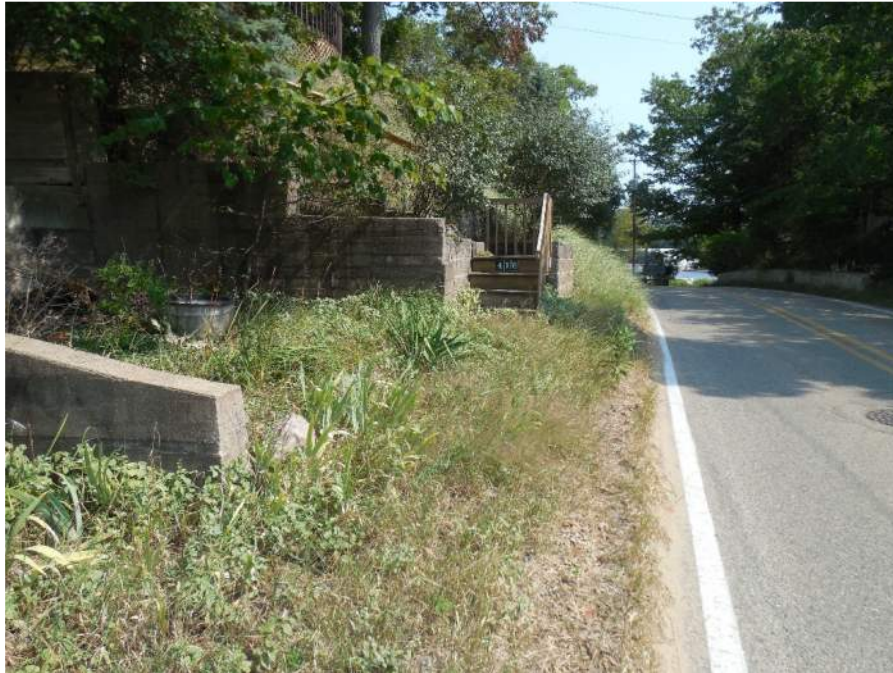
Photo 23: Retaining wall and stairs at 416 Park Street
