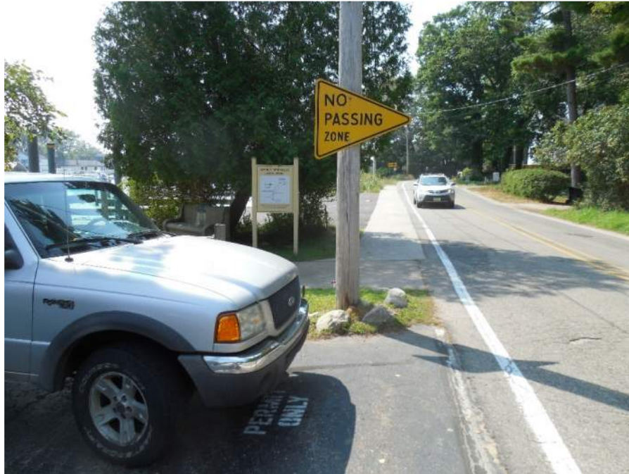
Photo 35: Utility pole at chain ferry, 3' clear from edge of asphalt Solution:
