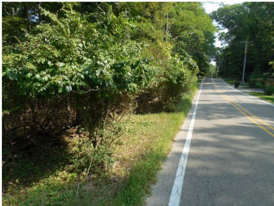
Photo 8: Brush between Lakeview Street and 71 Park Street and grade drop-off
