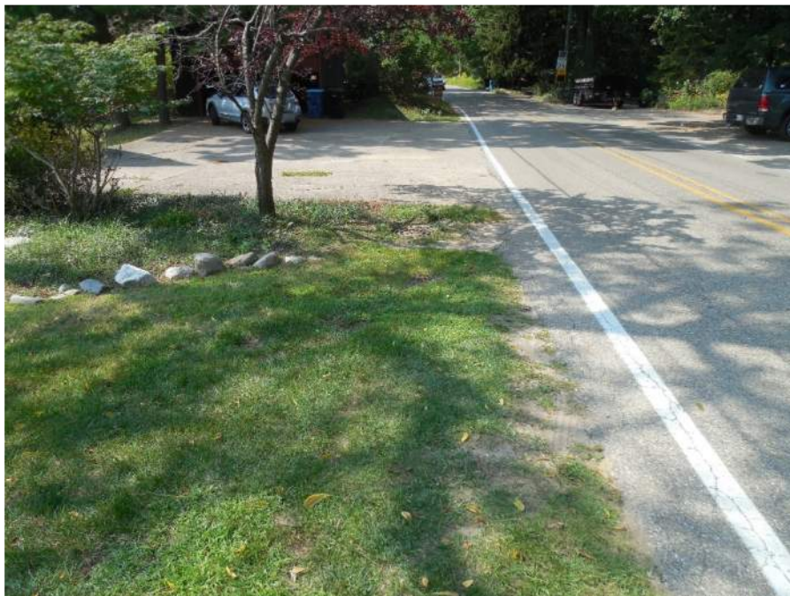
Photo 42: Catch basin south of 347 Park Street
