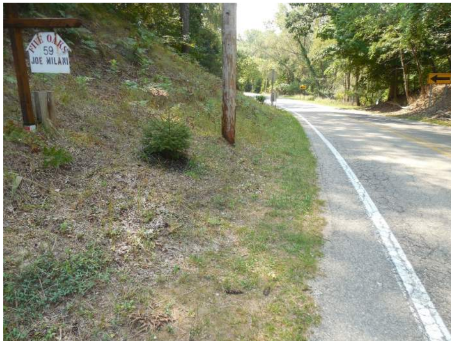
Photo 50: Slope south of 59 Park Street, utility pole is 5'+ clear from edge of asphalt
