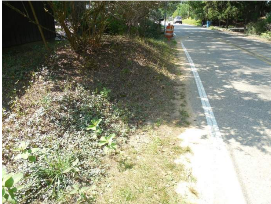
Photo 43: Slope across from 306 Park Street
