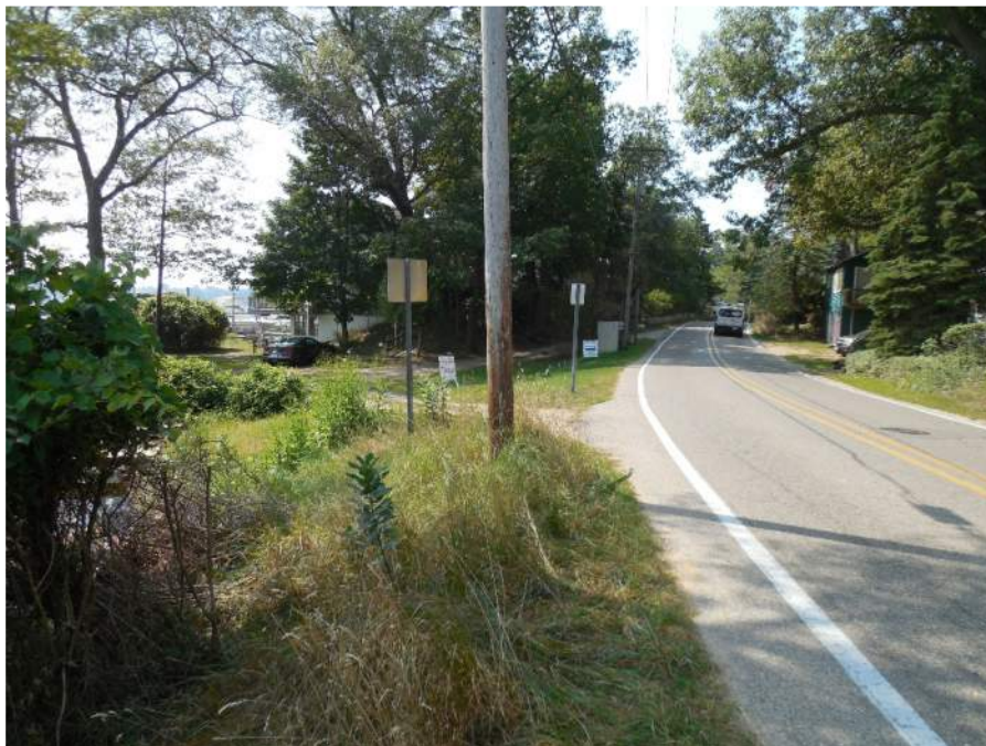
Photo 38: Utility pole across from 434 Park Street, 3' clear from edge of asphalt
