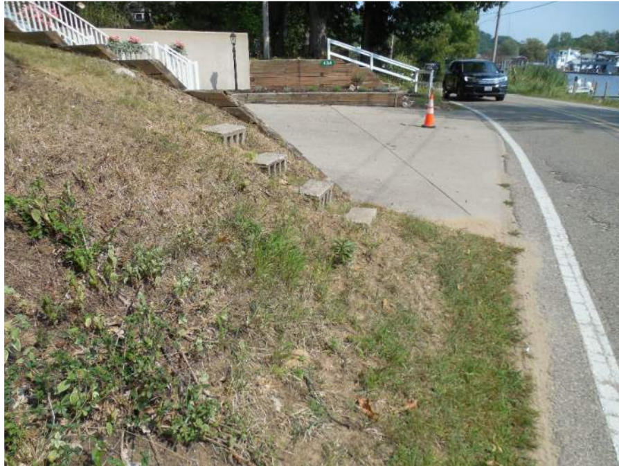
Photo 27: Slope and steps at 434 Park Street, south side of driveway
