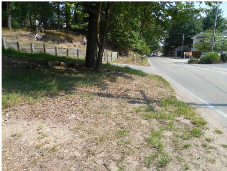
Photo 16: Slope at Vine Street – note: slope of Vine Street prevents meeting ADA guidelines for cross slope
