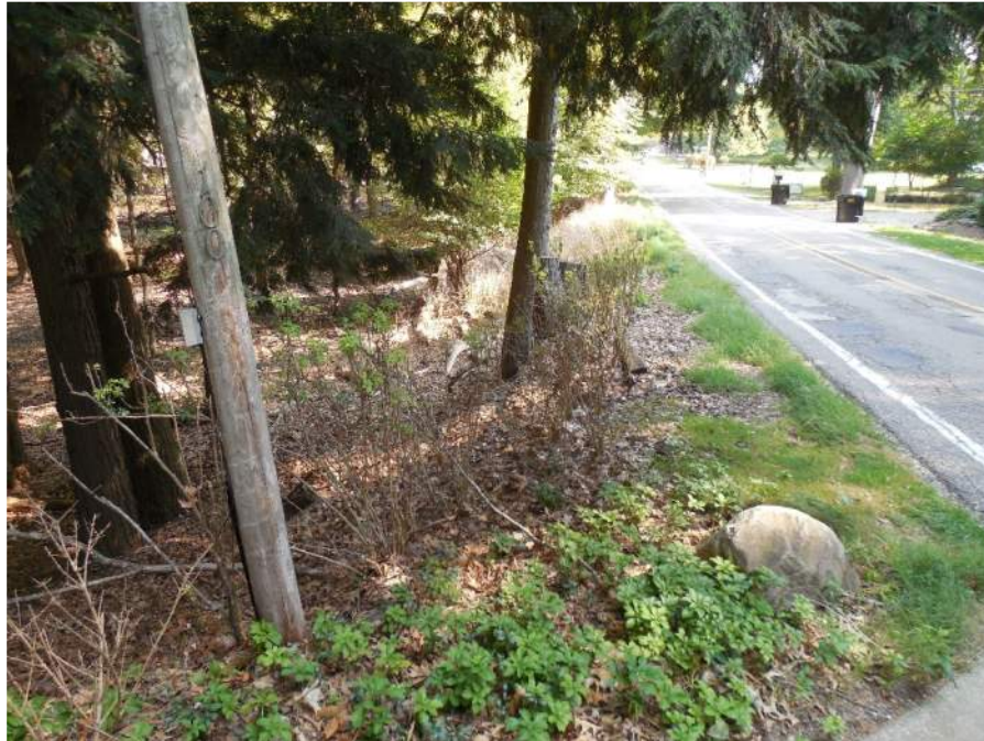
Photo 11: Trees, brush and grade drop-off north of 100 Park Street
