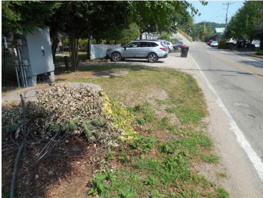
Photo 31: Lift station south of Perryman Street
