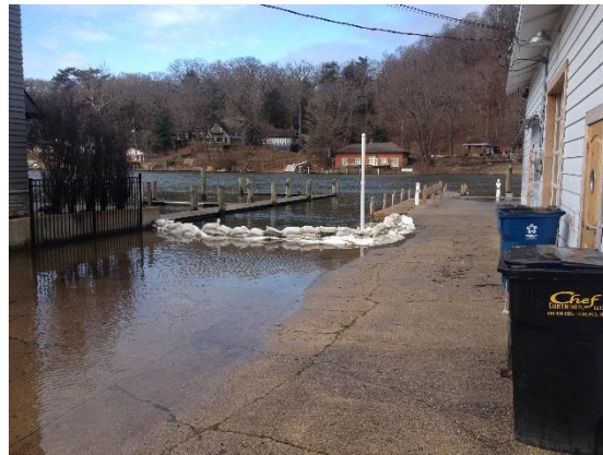
Figure 29 – Sandbags at driveway S. of Old Boat House
