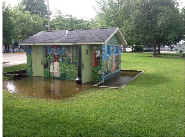
Figure 11 – Restroom looking southeast
