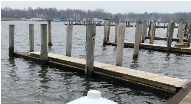
Figure 1 Existing Dock with new dock on top
