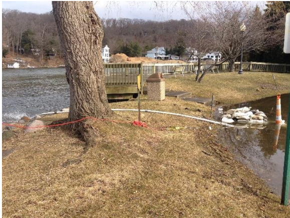
Figure 28 – Sandbags, sump pump and discharge
