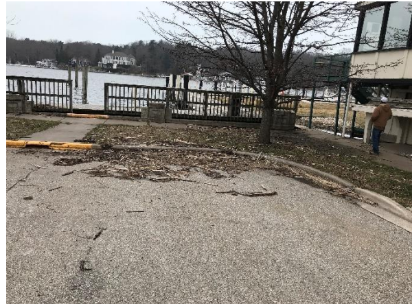
Figure 8 - Mason St Looking northwest
