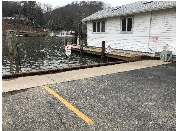
Figure 15 – Adjacent parking and sidewalk settlement
