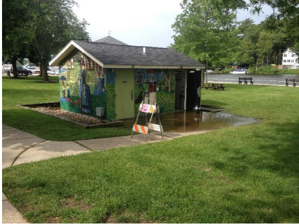
Figure 10 – Restroom looking southwest
