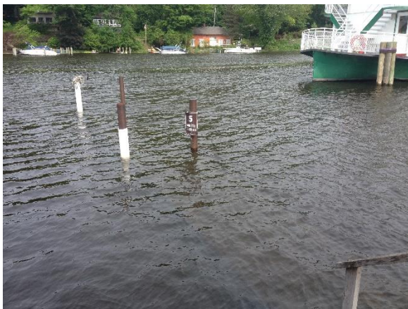
Figure 18 –Feb 24, 2020 submerged fixed dock
