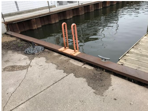
Figure 14 – Boardwalk settlement
