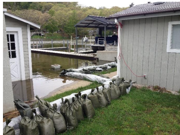
Figure 30 - Sand Bags and sump pumps at cottages Figure 31 - Sand Bags at river behind cottages
