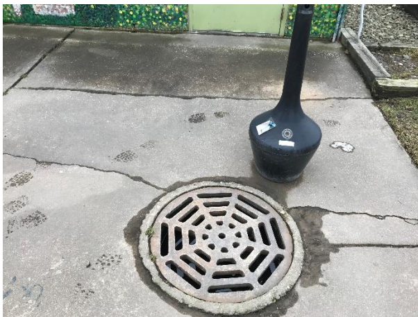
Figure 12 – Catch basin at entrance
