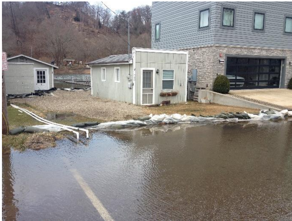
Figure 30 - Sand Bags and sump pumps at cottages Figure 31 - Sand Bags at river behind cottages
