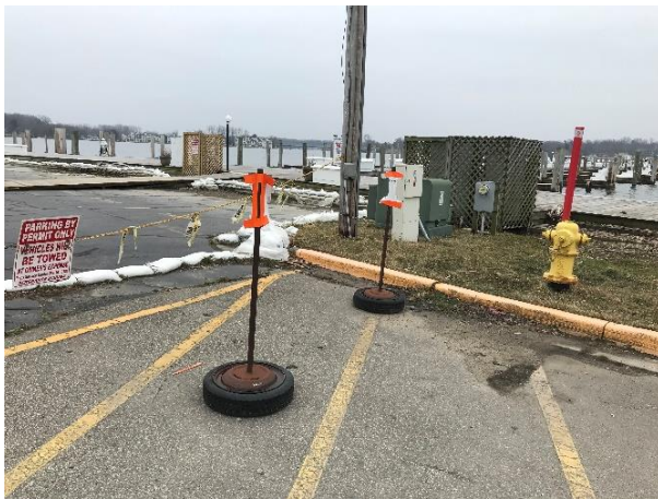
Figure 3 – Sergeant Marine Parking Lot
