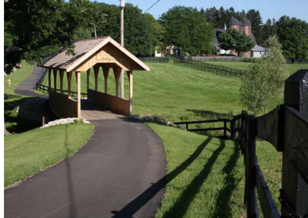
Covered Bridge on Grand River Drive
