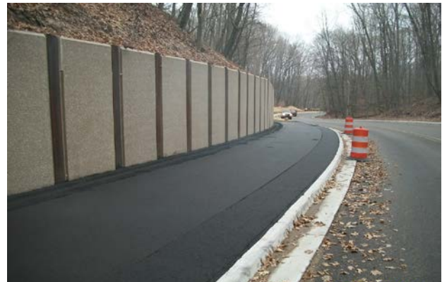
Soldier Pile Retaining Wall – Spring 2015
