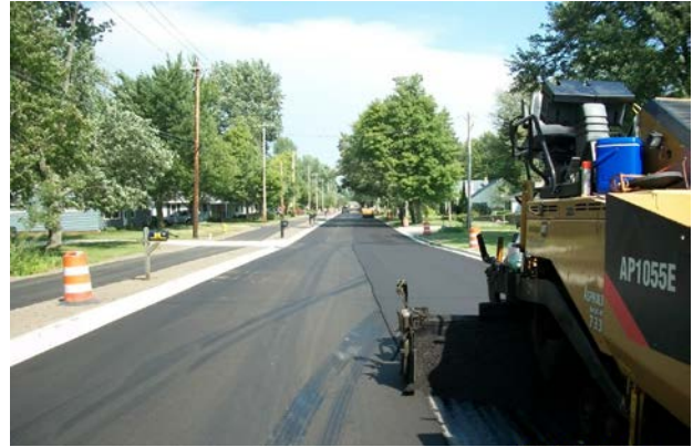
North Shore Road – June 2015
