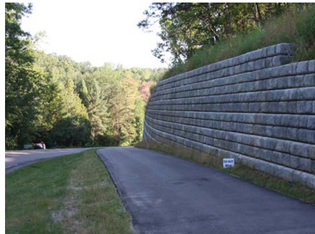
Retaining Wall on Grand River Drive
