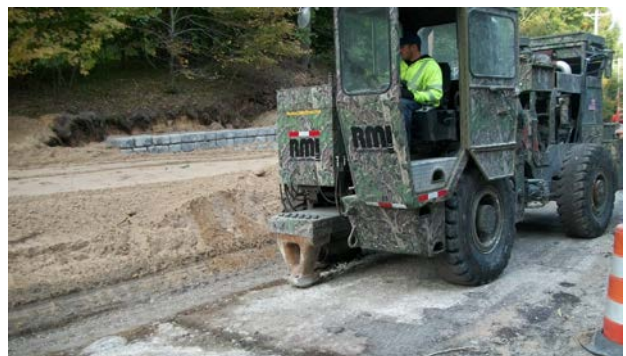
Rubblized Concrete – September 2014
