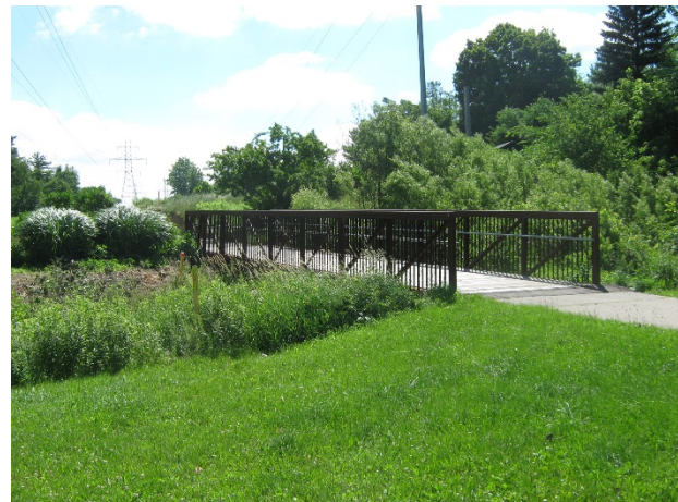
Bridge near Fuller Avenue
