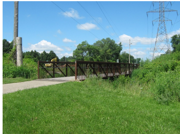
Bridge & Stream Crossing near Aerial Towers
