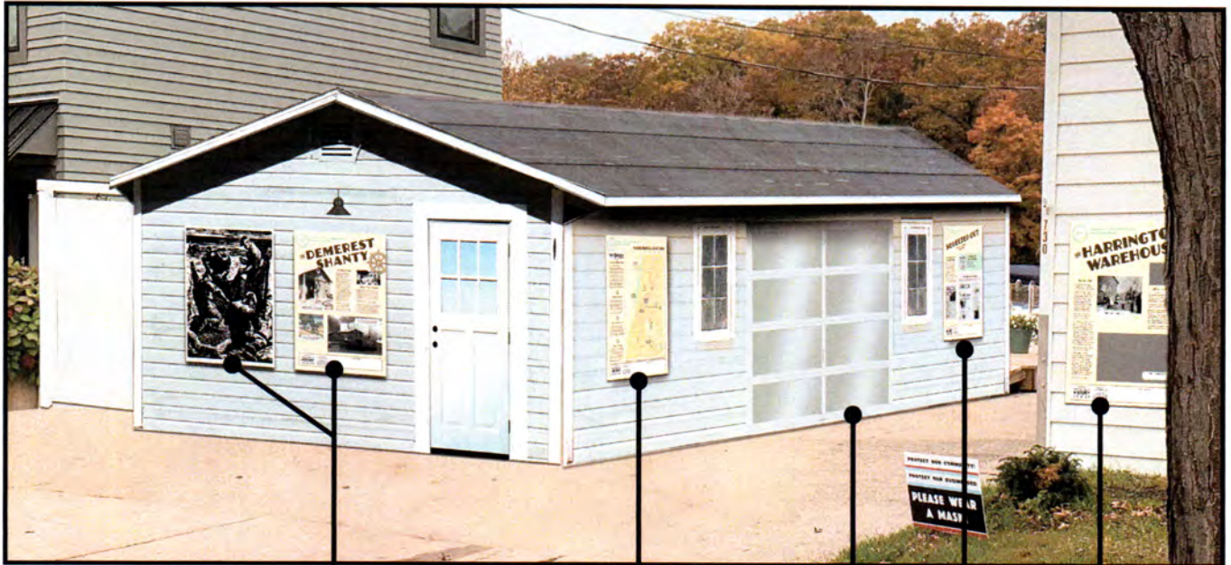
Building footprint approx. 14 x 26 feet
