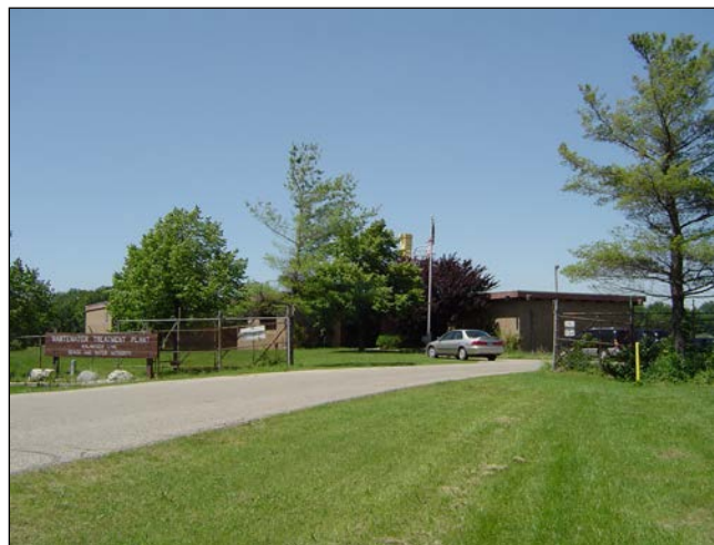
Photo 6-1 Waste Water Treatment Plant
