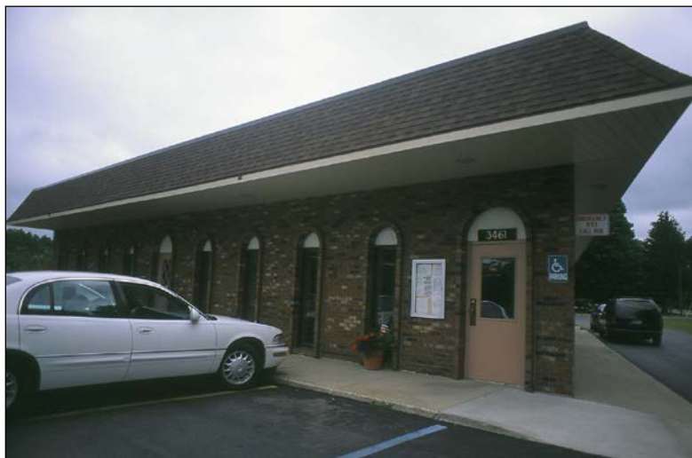
Photo 6-9 Saugatuck Township Hall
