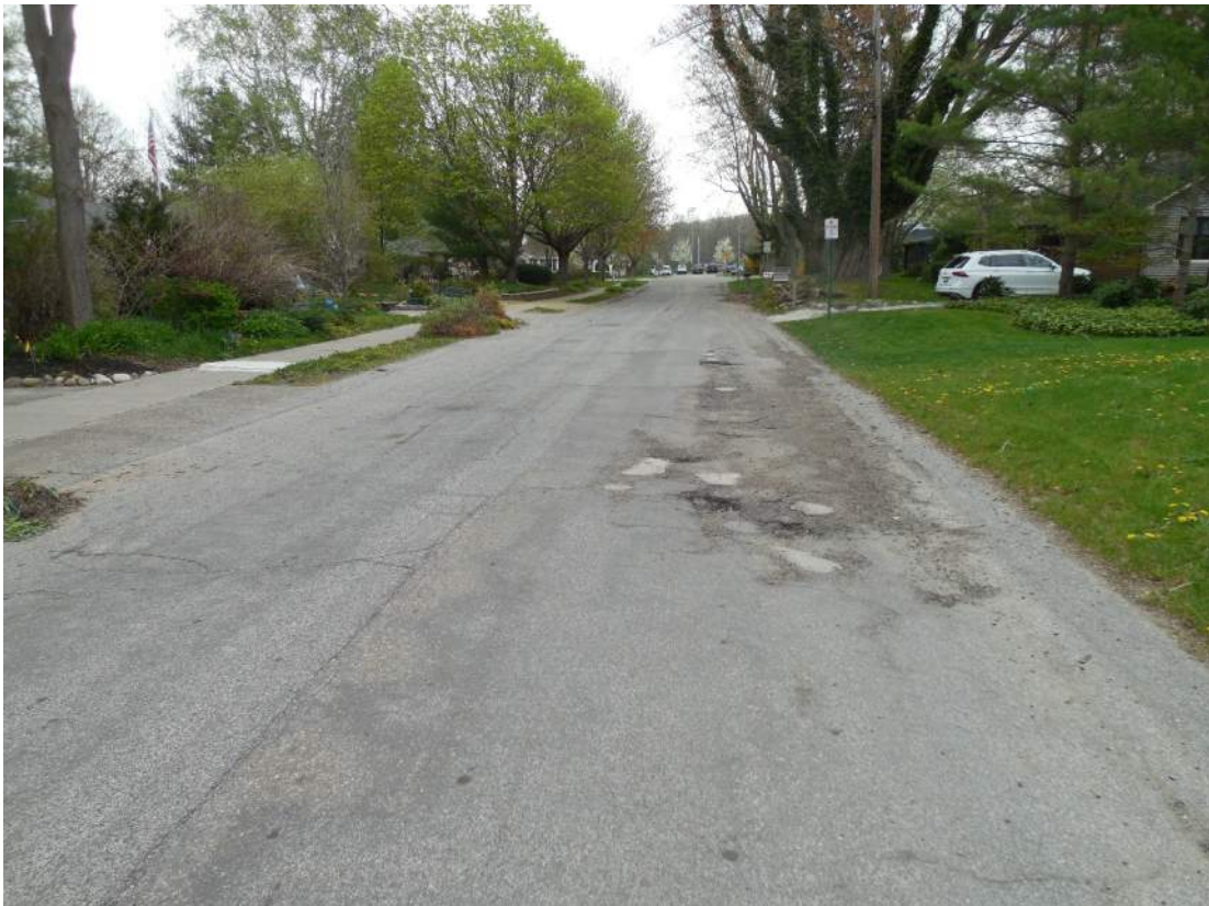
Hoffman Street west of Elizabeth Street looking east
