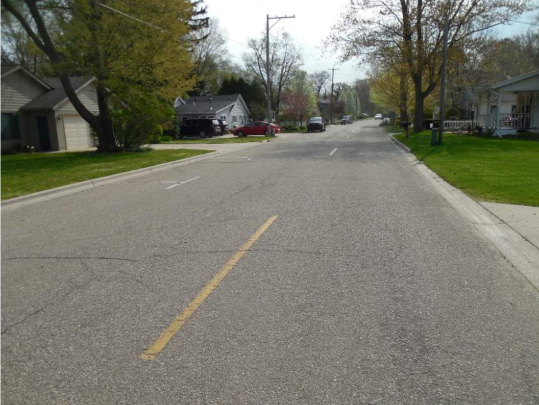
Lucy Street east of Butler Street looking east
