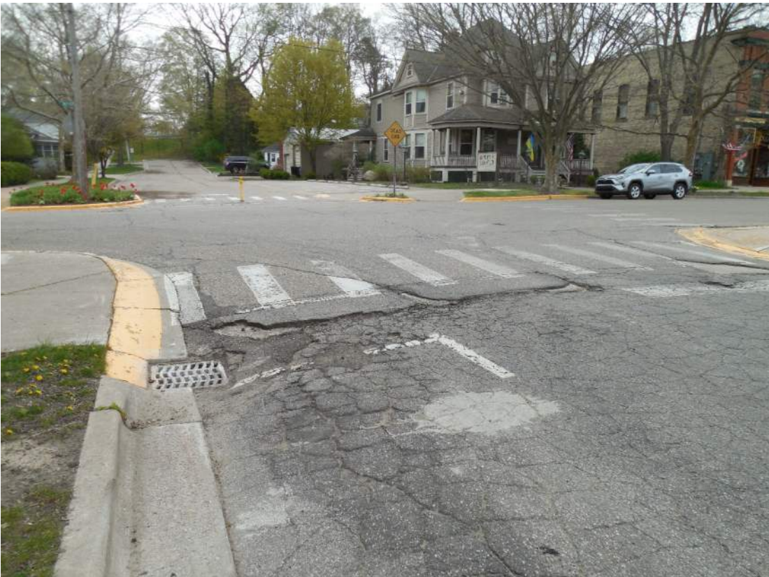
Mary Street looking southeast at Butler Street intersection
