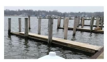
Figure I Existing Dock with new dock on top
