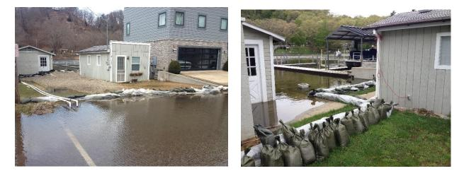
Figure 30 - Sand Bags and sump pumps at cottages Figure 31 - Sand Bags at river behind cottages
