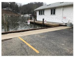
Figure 15 – Adjacent parking and sidewalk settlement
